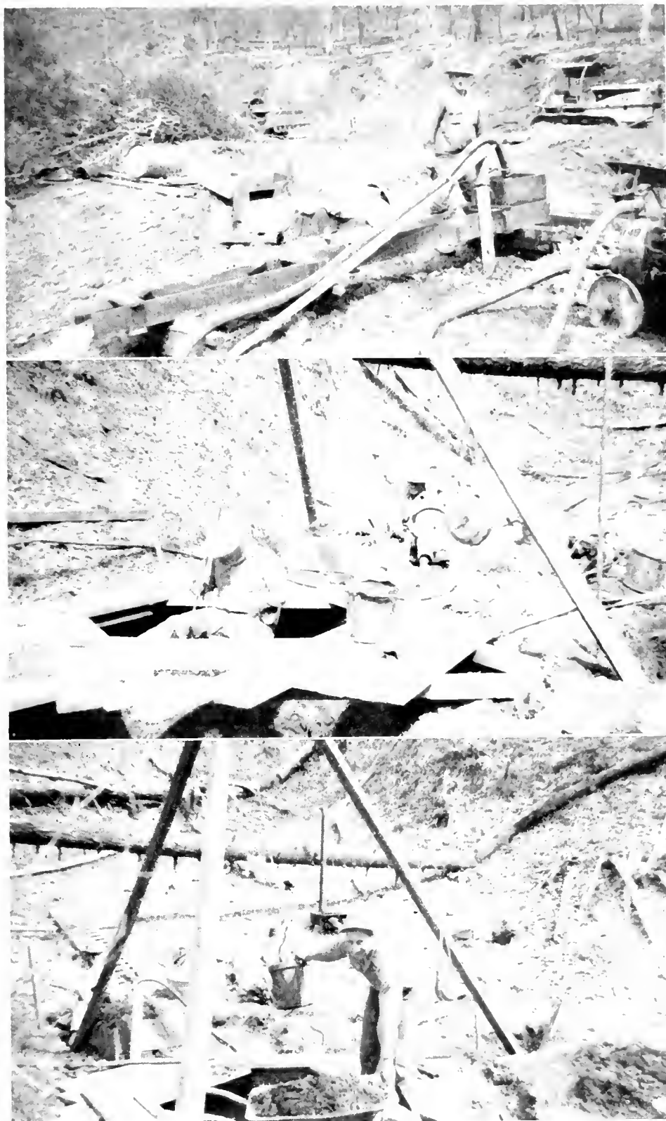
UPPER—Jib operating sluice box. Note clearing operations in background. CENTER—Jae on his way down. "Smooch" operating the air hoist. LOWER—Bill handling the bucket line.
